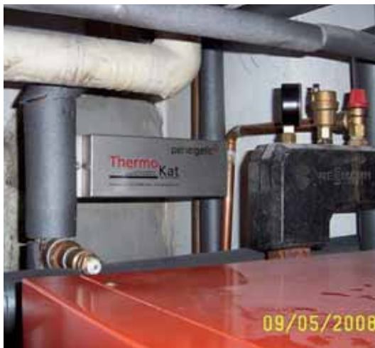
ThermoKat installation on the heating pipes directly after the boiler
