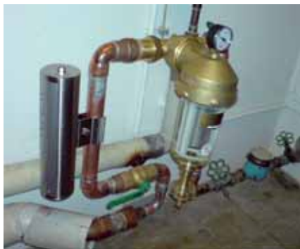
Installation of AquaKat L on cold water pipe after back-washing filter
