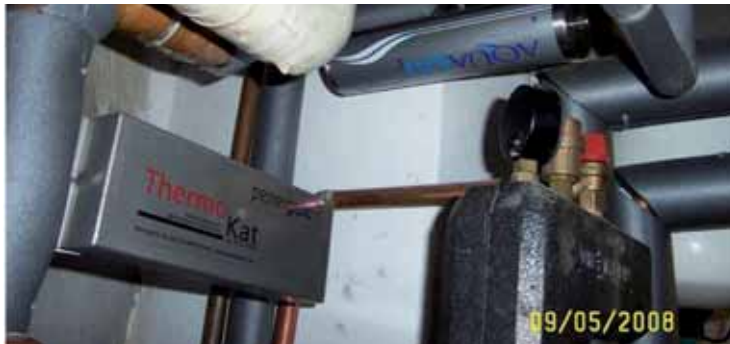
Additional installation of Aquakat L for revitalisation on warm water pipe after water heating device (top of picture)
